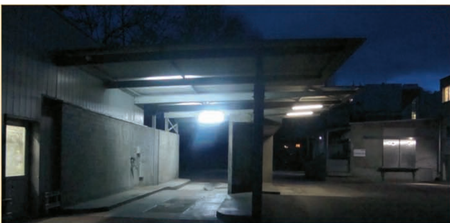
The luminous effect of the newly installed LED tube at the outdoor washing area can be seen clearly (left rear). Marco Egli explains: "Here one can see the difference between conventional lights and LED tubes very clearly, and the light quality is extremely good!" (Photo: Marco Egli, ZSHAG)
